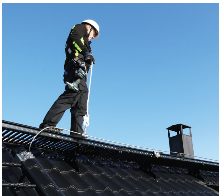
Pisko SafeLine and Pisko rope fastener are complementary solutions. Pisko SafeLine wire system is a fall arresting safety rope anchoring point primarily recommended as part of access ways. Rope fastener attached to a walkway enables better maintenance work in the danger zones of the roof with the user attached to a safety rope.
