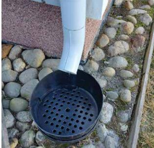
The same black plastic rainwater drain basket is shown, but it is empty and clean, with a perforated bottom. The white downspout pipe is visible and clear. |
