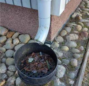
A black plastic rainwater drain basket is shown, filled with a thick layer of brown leaves and twigs, completely blocking the opening of the white downspout pipe. |
