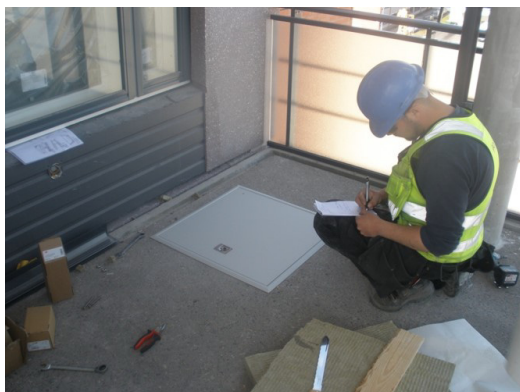
Emergency exit hatch installed
