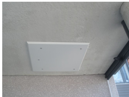
Emergency exit hatch from below
